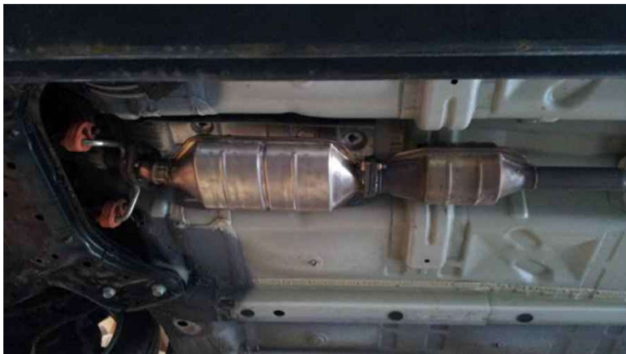
Figure 6 Ammonia Emission Reduction System
