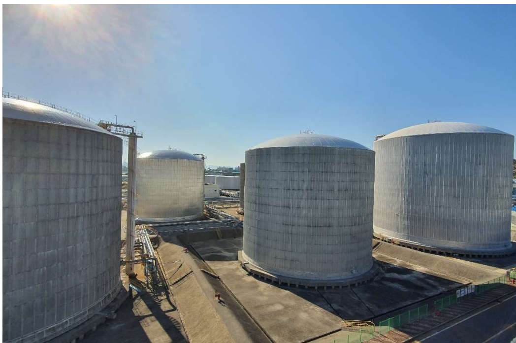
Figure 5 Ammonia Storage Tank <Source: LOTTE FINE CHEMICAL >
